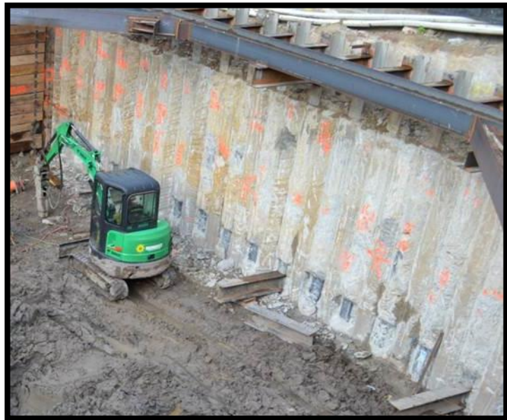
Figure 4.1 – Secant Wall | Courtesy of DAVIS
