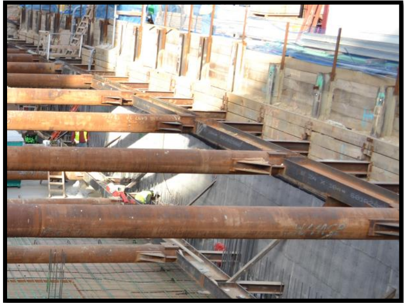
Figure 3.1 - SOE System | Courtesy of DAVIS
