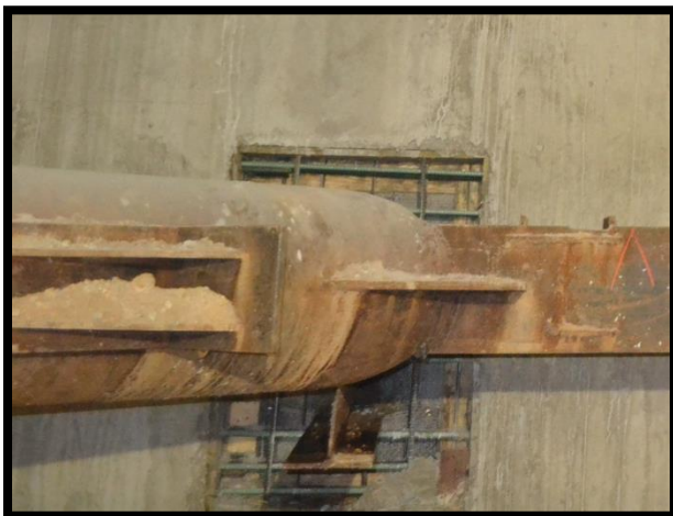
Figure 3.2 – Formed Tie-in | Courtesy of
